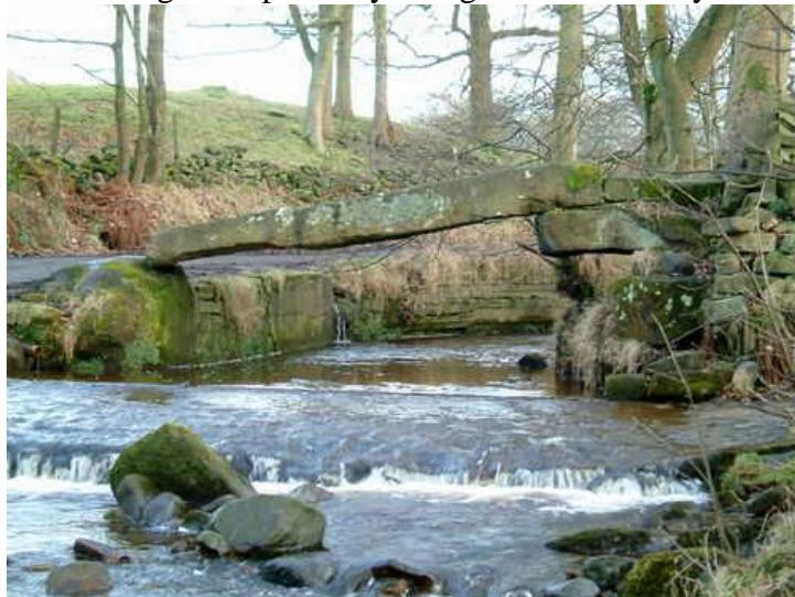
Haworth. It is a unique single-span bridge crossing the banks of the beck. You can see from the photograph the the bridge rests precariously on the edge of a natural rock outcrop. Yvonne is standing on a system of huge balance stones that support the main Clam bridge. Clam Bridge is believed to be the oldest bridge in the Wycoller area- perhaps dating back to Bronze-Age times. Perhaps as old as Stonehenge!
